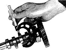
MEASURING INJECTION PUMP CAMSHAFT LOBE
